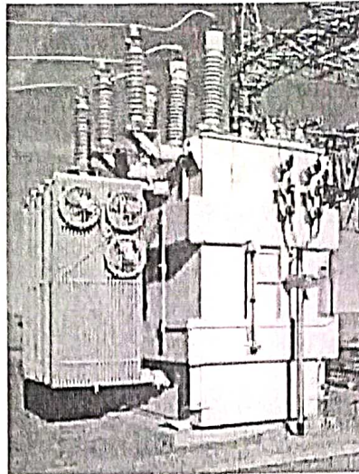
Fig 2.4 Auto Transformer
