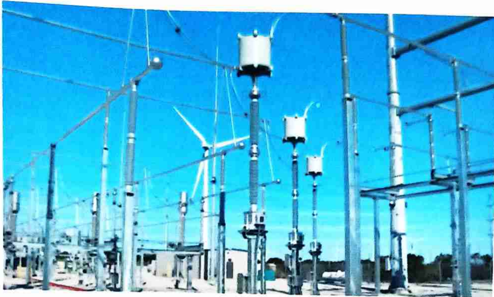
Fig:- WAVE TRAP
