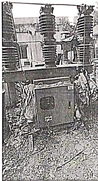
Fig:- VACUUM CIRCUIT BREAKER
