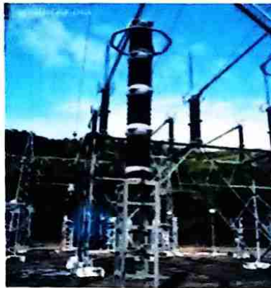
Fig:-LIGHTNING ARRESTER
